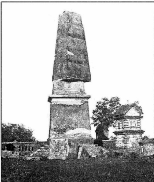
Figure 1 Rotation of the monument to George Inglis (erected in 1850 at Chatak, India) as observed by Oldham (1899) after the 1897 Great Shillong earthquake. This monument had the form of an obelisk rising about 20 m high from a base 4 m on each side. During the earthquake, the topmost 2 m section was broken off and fell to the south and the next 3 m section was thrown to the east. The remnant is about 6.5 m in height and is rotated about 15^\circ relative to the base. Such rotations can be due to strictly translational accelerations and don't necessarily require rotational ground motion (see text).
